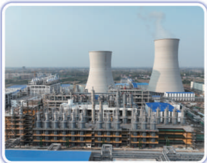
Jindadi Group CHP 3×390 t/h
